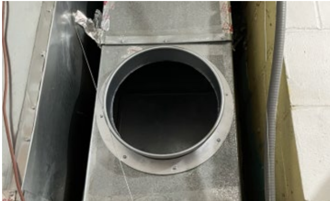
Prep the ductwork & registers
